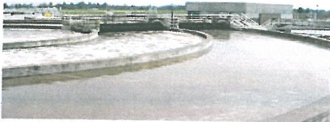
Orbal Multichannel Oxidation Ditch for Wastewater Treatment
