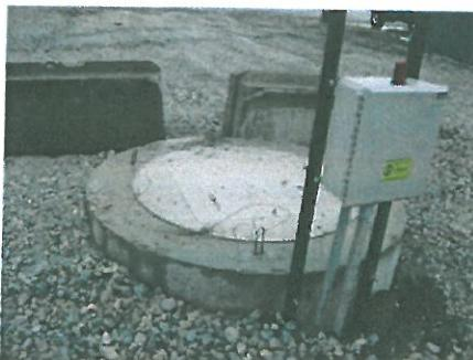
Sewage lift stations/pump stations may be used as a matter of economics or to overcome inadequate hydraulic head when it is obvious that no other solution is practical. For instance, it may be more economical to utilize a sewage pump station to pump or lift the sewage over a ridge and let it flow by gravity.
