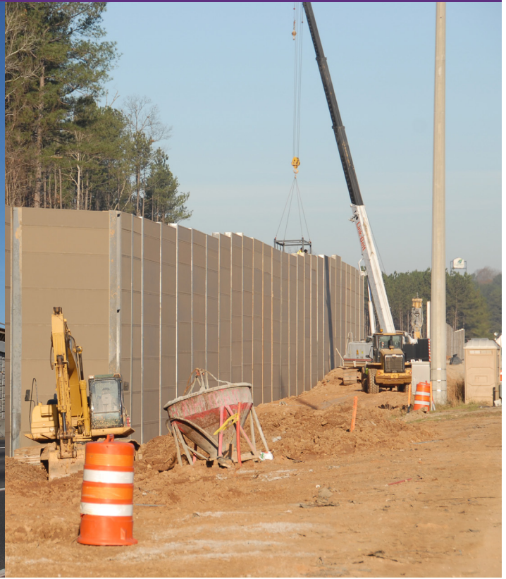
Sound wall construction on the southbound section at Walt Stephens Road
