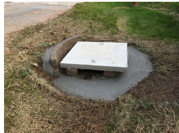
Harkins Street- Drainage Ditch and Catch Basin Repair
