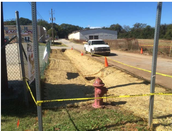
Harkins Street- Drainage Ditch and Catch Basin Repair
