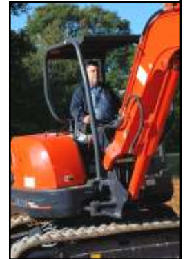
Water Distribution employee J. R. McMahan puts the new Kubota mini excavator through its paces.
